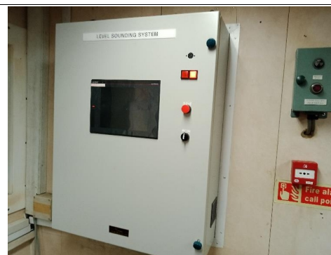
17) Newly fitted ballast tank level monitor.
