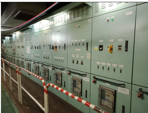
20) Switchboard in machinery space.
