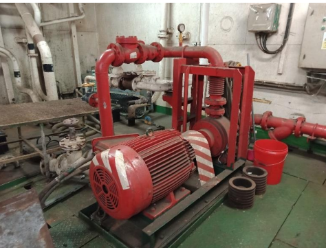
27) Fire pump in machinery space.
